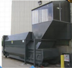
Full Enclosure SC Compactor Installation
